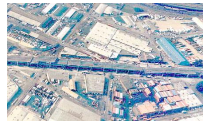
g / The collapsed section of the Nimitz Freeway.
