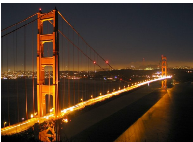
The Golden Gate Bridge's roadway is held up by the tension in the vertical cables.
